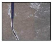
Prime Crack With Quick-Repair 15
