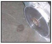
Clean Crack With Diamond Saw Blade
