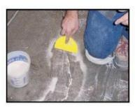
Fill Crack With Silica Sand
